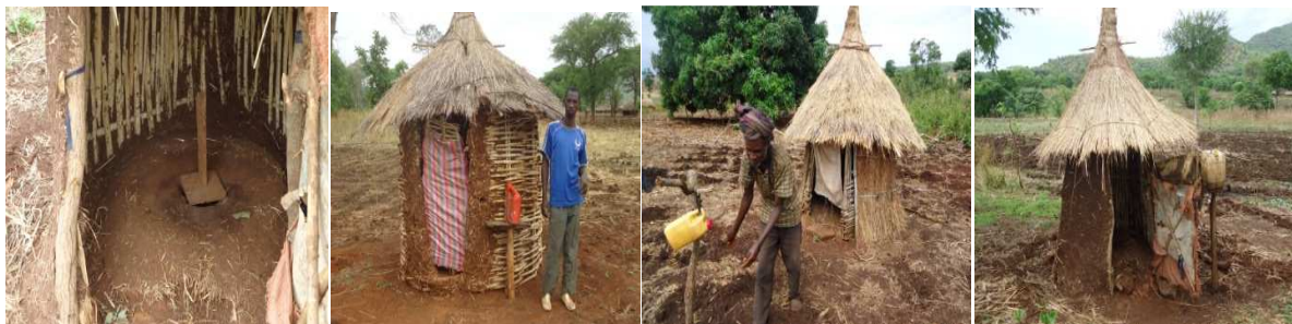
Picture 2: Some of the Private Pit Latrines constructed in the Target Communities
