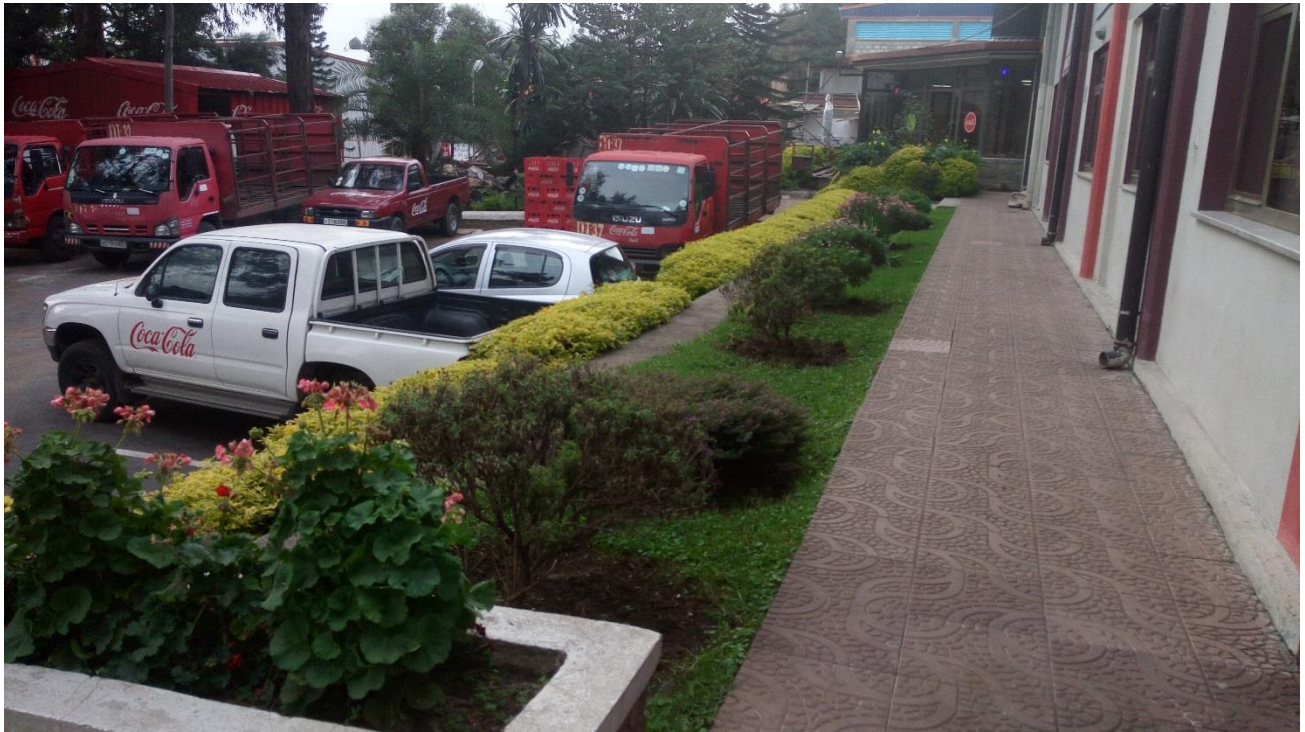
Picture 6 Clean Compound, In front of Administrative Office Building
