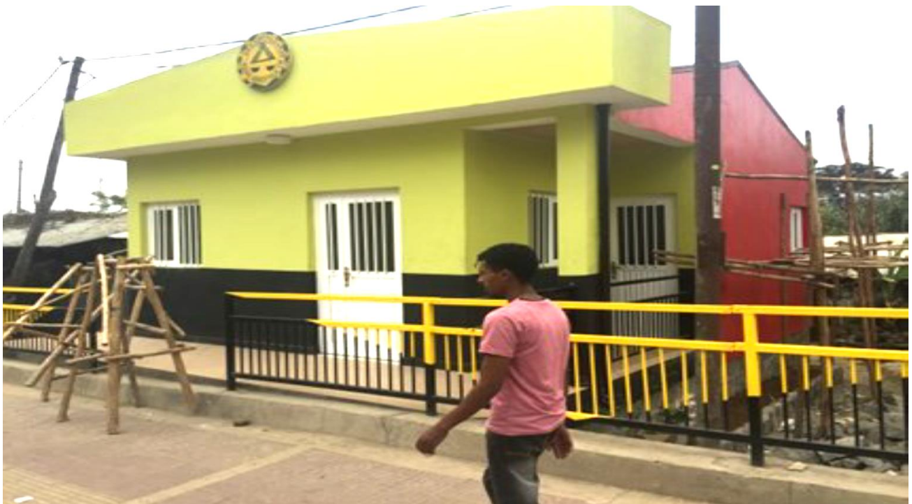
Picture 10 a community Police Station constructed by EABSC/Coca-Cola
