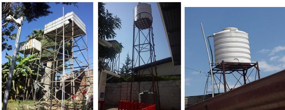
**Figure: 4. 6 Common Ways of Placing House Hold Water Storage Tanks.**
