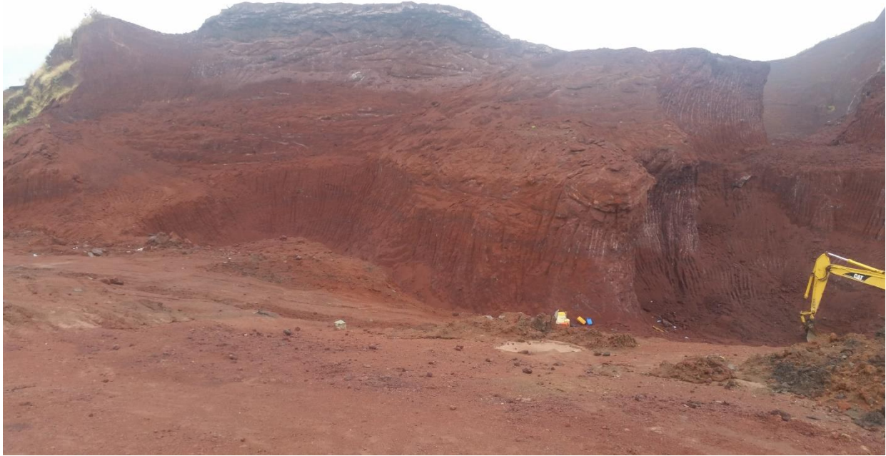
Figure 4-3 Degraded Borrow pit land around Dukem
