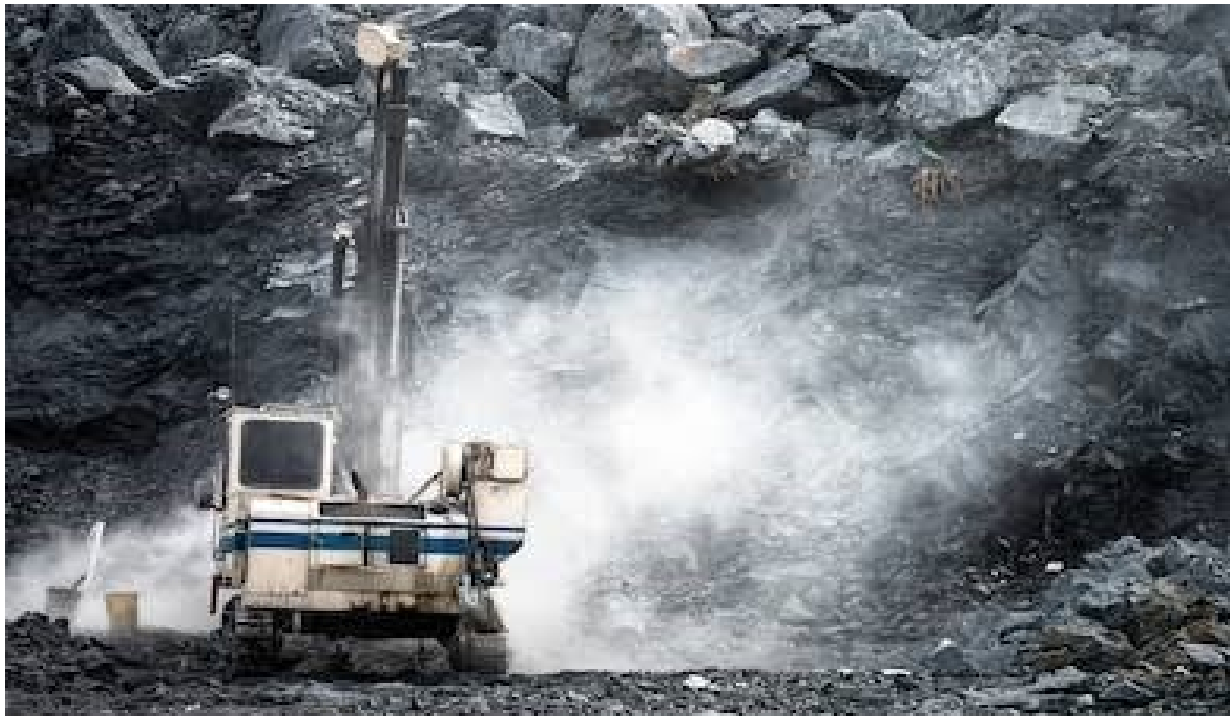
Fig. 4.3 drilling activity in Wollenchity quarry site
