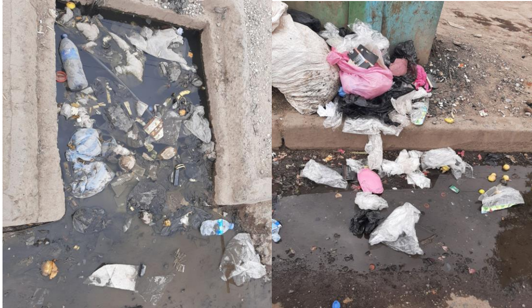
Figure 2 Waste plastics blocking urban sewerage system, Addis Ababa, Jemo Area
